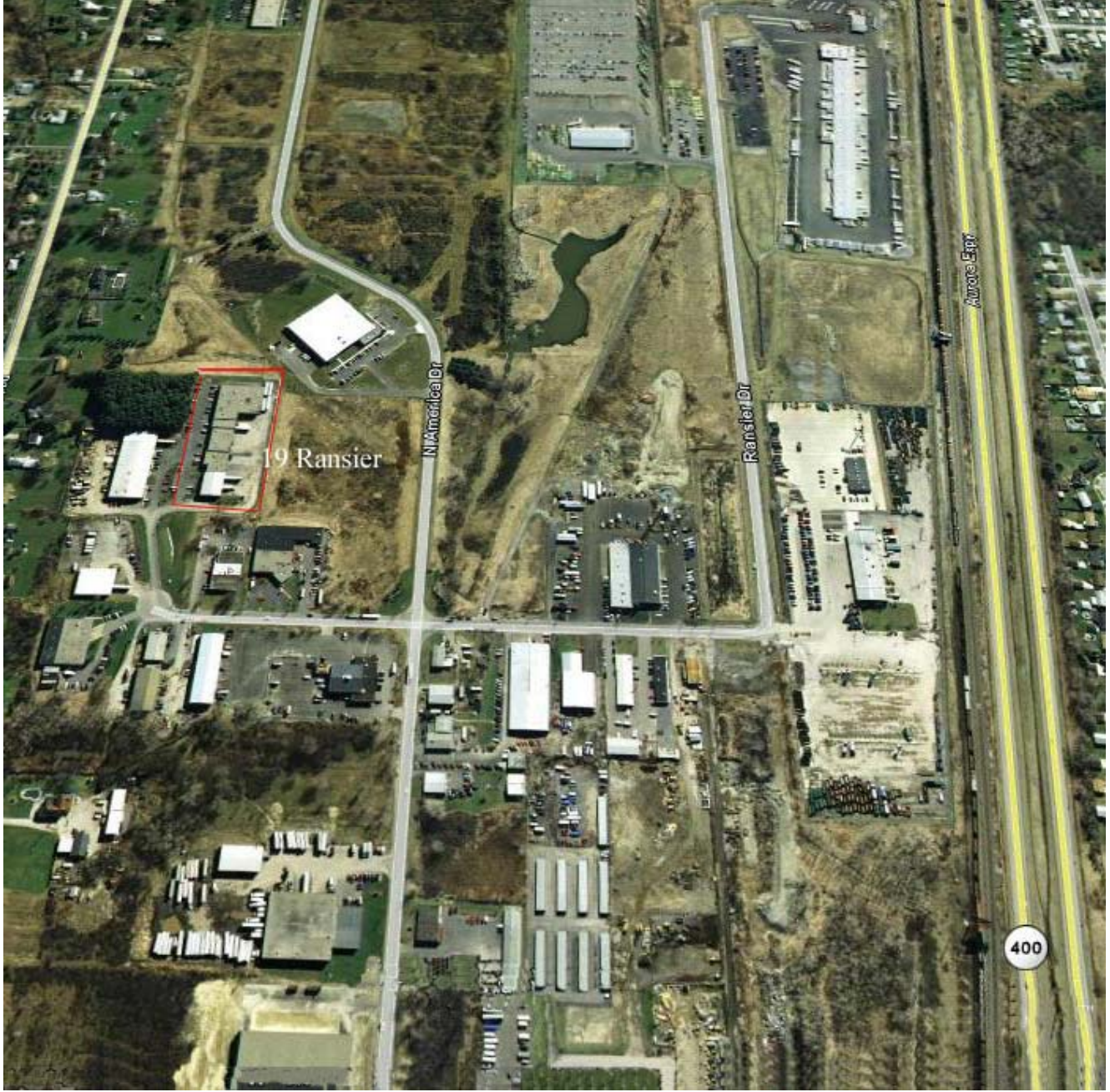
Aerial View of Ransier Commerce Center
